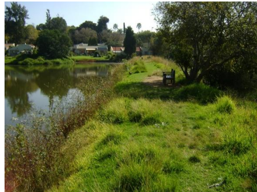
Looking west along the dam wall
