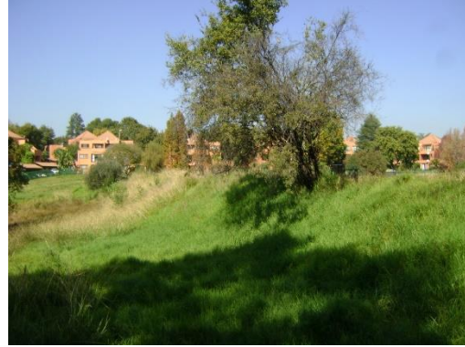
Downstream side of the dam wall
