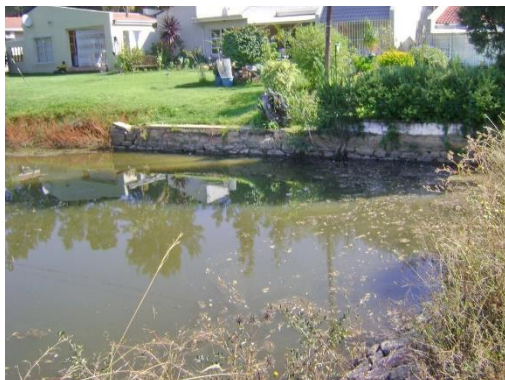
Spillway training wall, western side
