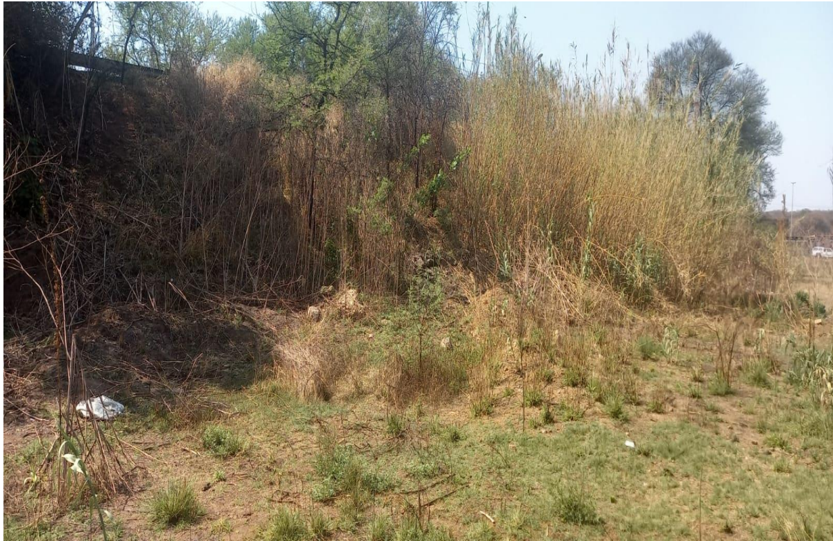
Figure 7: Some material of the soil might have moved downslope.
