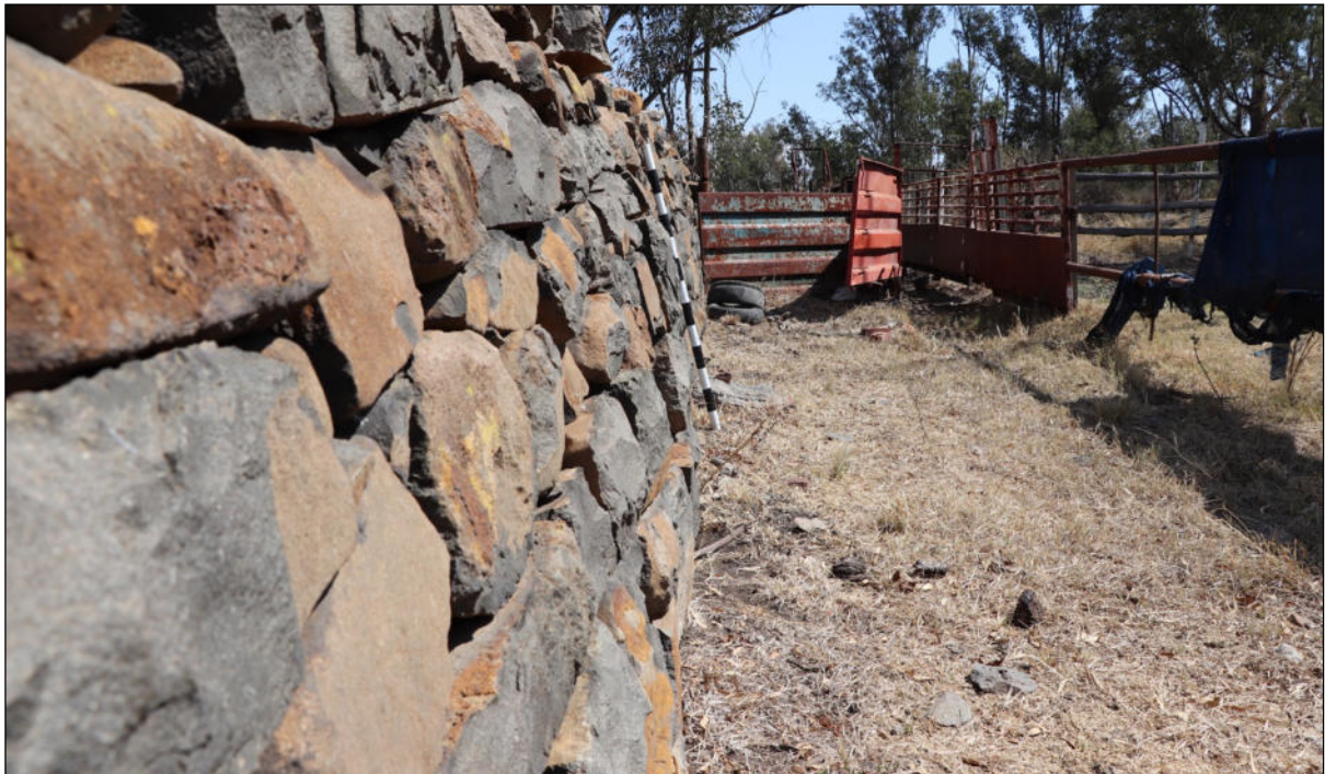
Figure 27 – This view along the inside wall of the original component of the livestock enclosure clearly depicts the battering that was built into the wall to increase its stability. This section of the livestock enclosure can be seen as the first building phase in its construction. Scale is in 10cm increments. Refer photographic reference P7 on map depicted in Figure 20.
