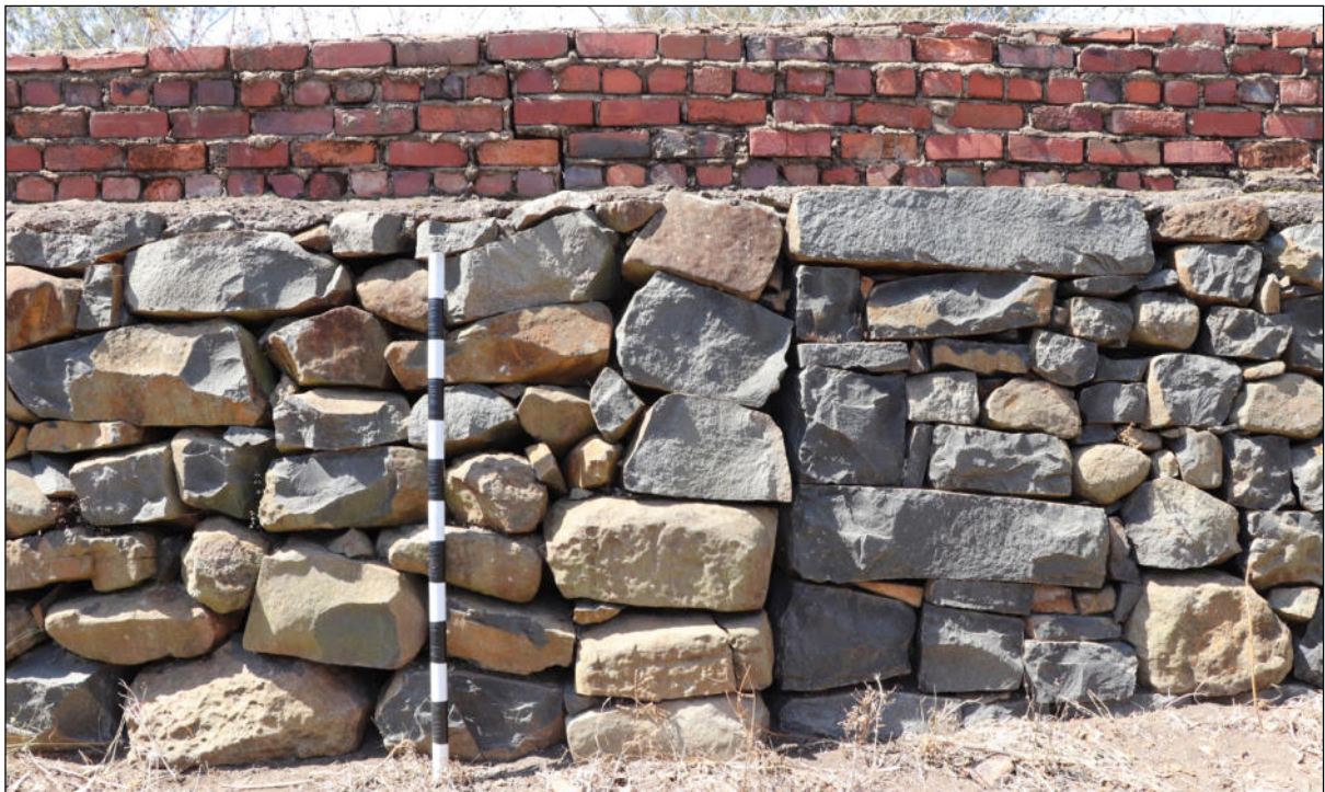
Figure 28 – Three building phases in the construction of the livestock enclosure can be identified on this image. The first building phase is represented by the stonewall on the right, with the second building phase represented by the stonewall on the left. The brickwork visible on top of both these stonewall sections, represents a third building phase. Refer photographic reference P8 on map depicted in Figure 20.
