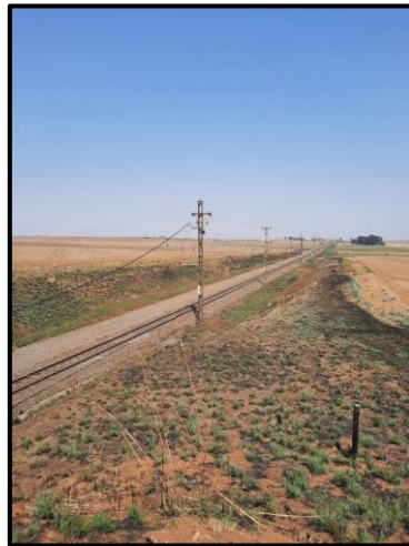
Figure 7.4. Railway infrastructure in the study area.
