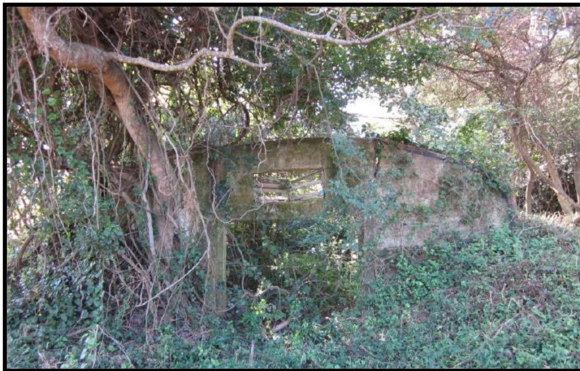
Figure 10. Entrance to southern Bunker from the south (Source: Whelan 2011).
