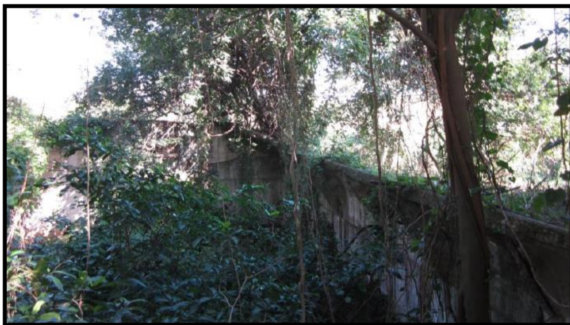
Figure 11. Southern Bunker from above (Source: Whelan 2011).
