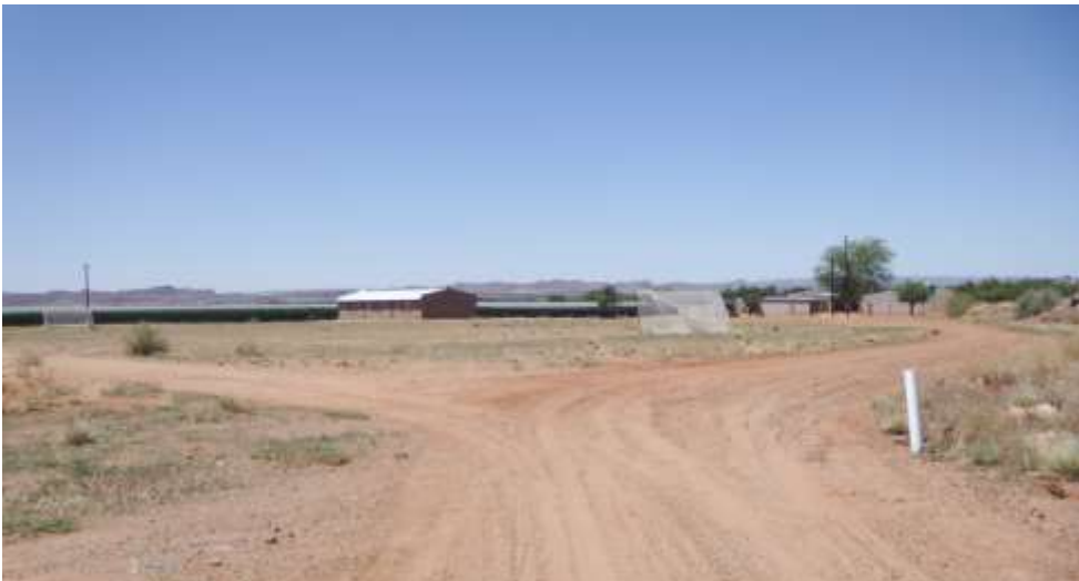
Figure 9 Structures and agricultural features associated with ongoing farming activities.
