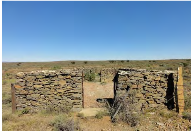
Figure 6.28: Dipping kraal: a low-walled rectangular structure made of local stone. It has two entrances, one leading to a small pool. Adjoining fences indicate its likely use as a dipping kraal. Graded 3c. GPS:32,56.9691S22, 36.9005E
