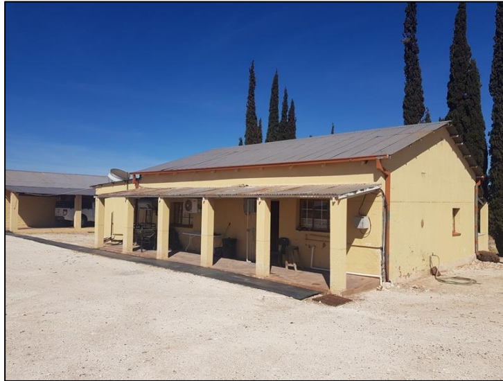
Figure 5-9: View of the Biesieputs farmhouse at Site Exigo-ZPM-CP03.
