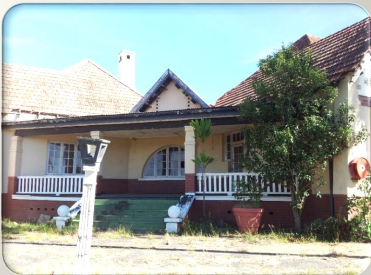
The existing small covered verandah to be increased in size. The new balustrade and brick work to match existing.
