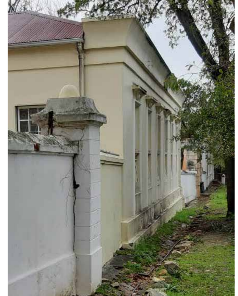
Figure 60. Government Avenue wall tying into the Egyptian Building.
