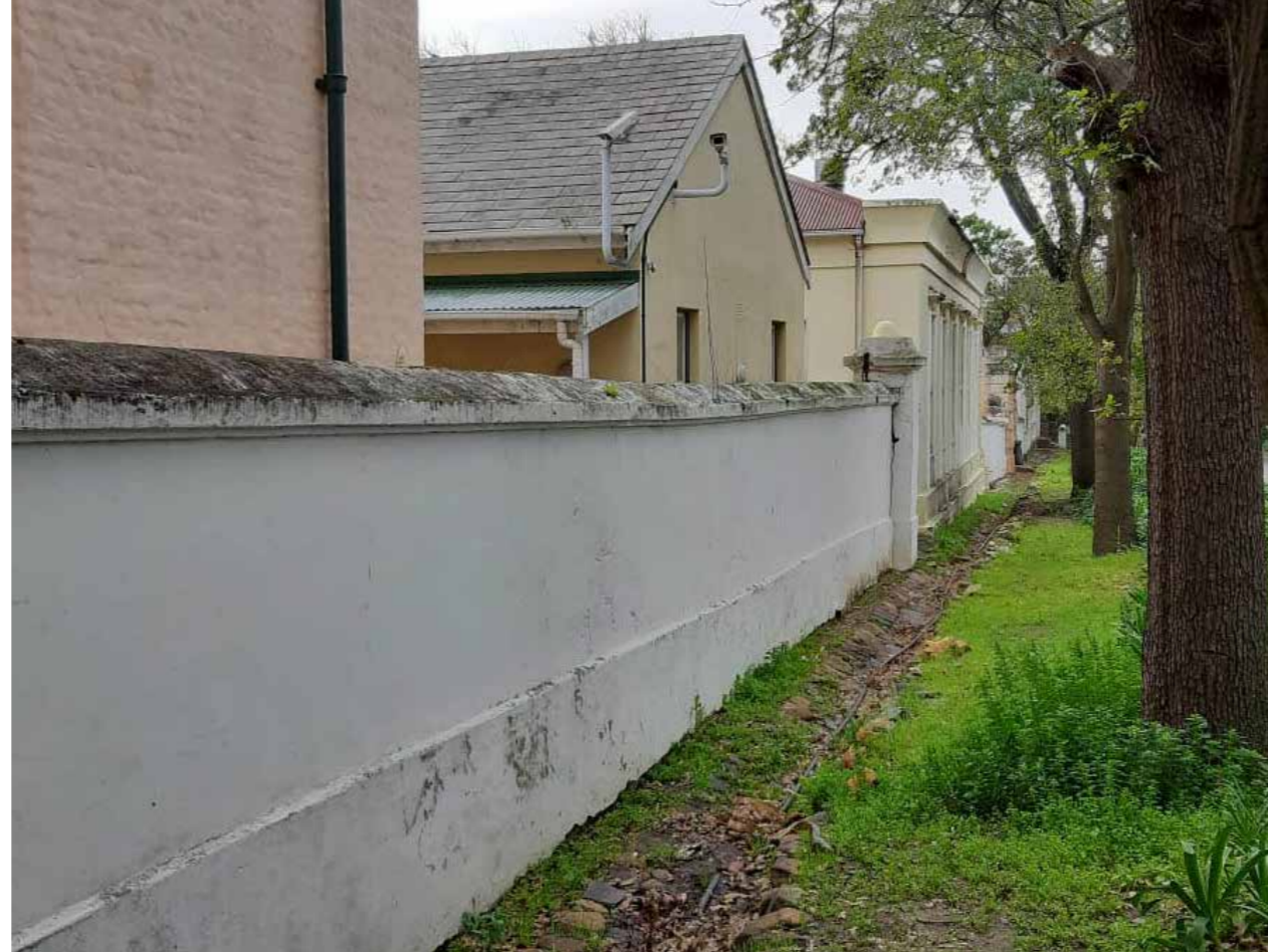
Figure 59. Government Avenue wall running along Hidding Campus structures.
