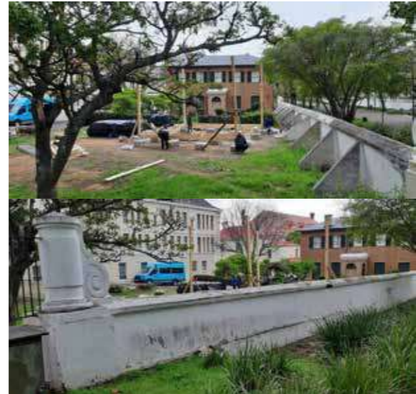
Existing boundary wall
