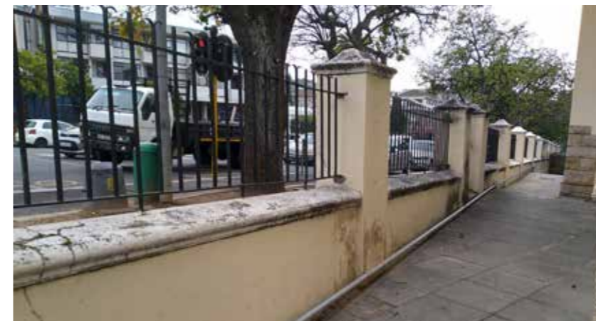
Figure 44. Existing Type 1: Boundary wall with wrought iron infill
