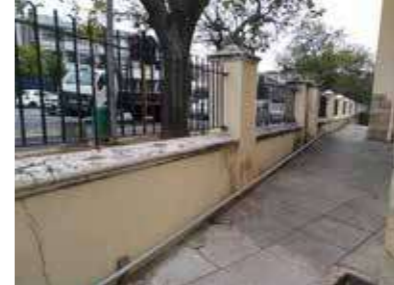
Existing boundary wall with fencing infill
