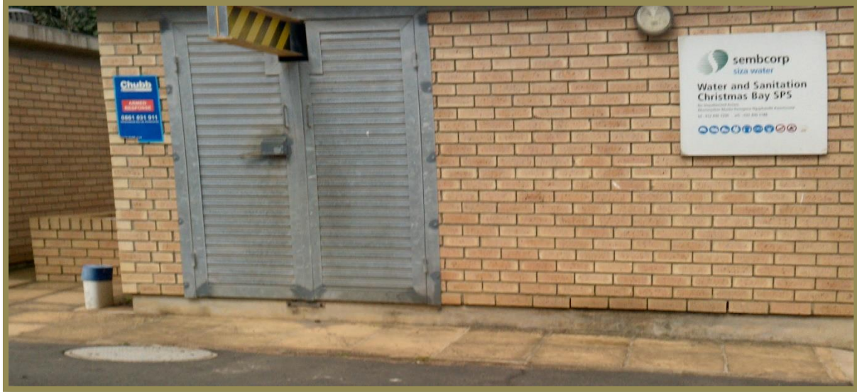
Figure 3 Existing Christmas Bay Pump Station
