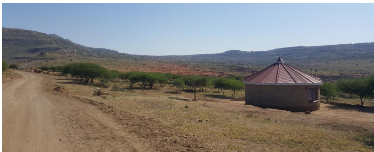
Figure 2 Proposed water reticulation pipes to be set along the existing road alignments
