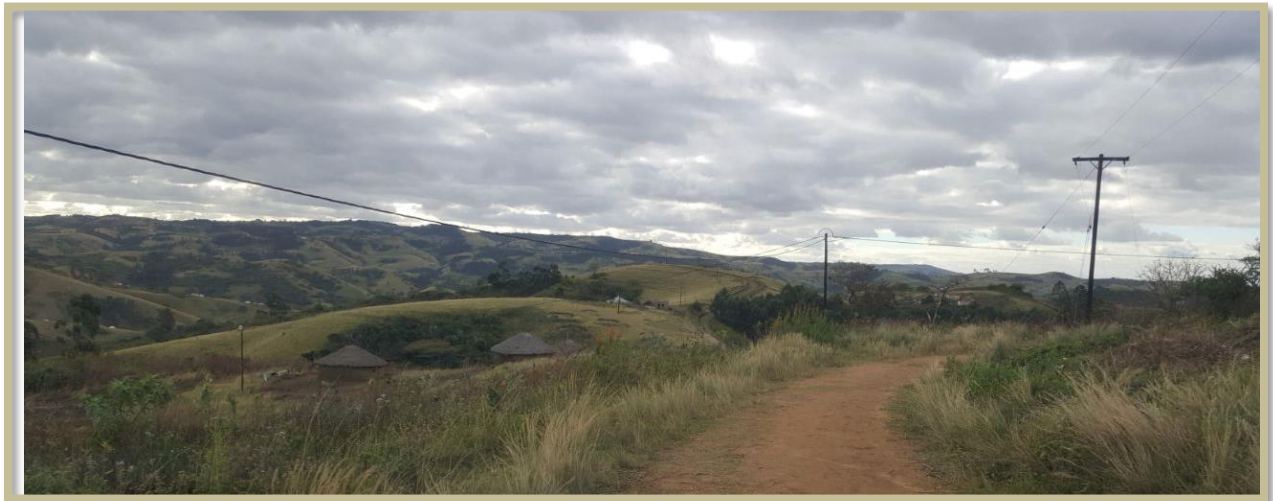
Figure 3 Abashumi access road in Ward 6 to be upgraded along existing roads and tracks
