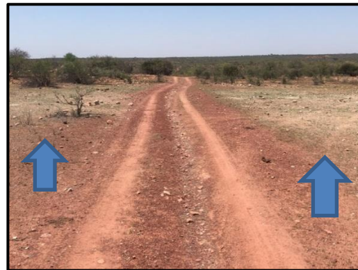
Figure 29: Existing access road cutting through vitrified dung deposits marking site 2229AD 208 on the right and site 2229AD 209 on the left.
