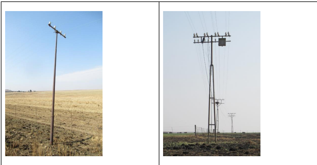
Figure 24. Old type metal telephone poles
