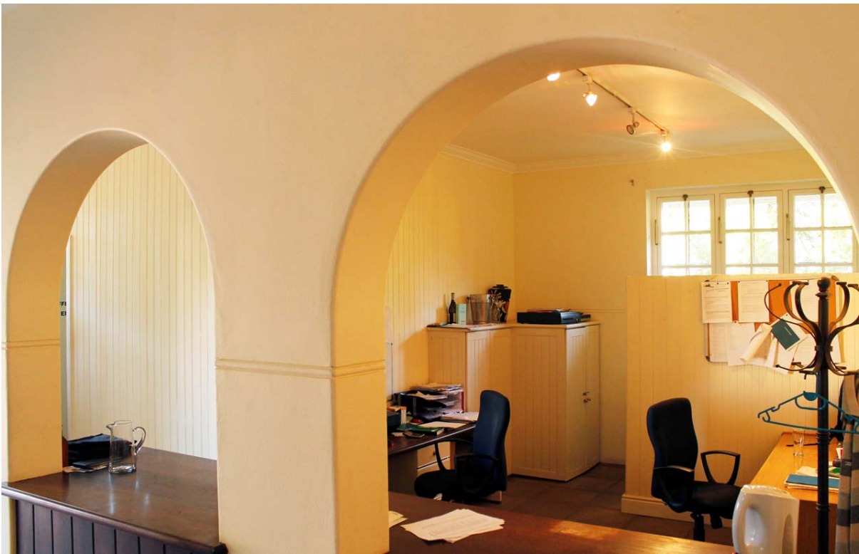
Figure 12: The existing office in the eastern corner of the building, which will be converted to accommodate a small office and toilets. The arches will be filled in and doors inserted. The outside windows will remain unchanged.
