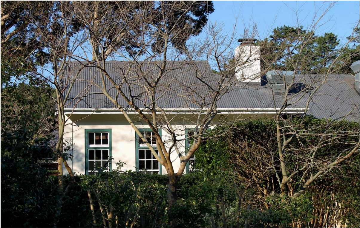
Figure 17: Outside view of the existing western wing. The second and third windows from the left will be replaced by French doors of the same height as the windows. This far end of the building is not visible from Spaanschemat River Road.
