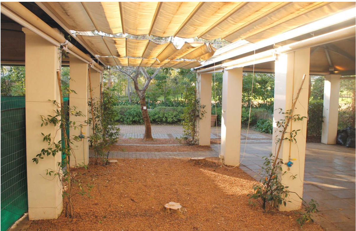
Figure 18: Current view of the courtyard at the back. The retractable cover that links the two hard canopies will be removed and the space in the foreground will become a glass-enclosed, flat-roofed wind lobby, using the existing columns.
