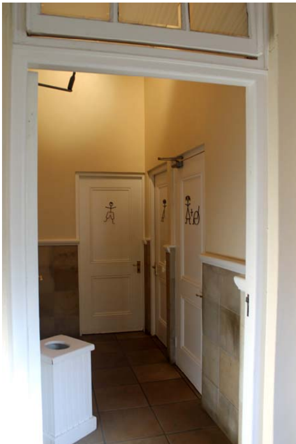
Figure 14: The existing toilets, built by Michael Dall Architects in 2008, which will be demolished and the space incorporated into the proposed open plan food hall. The toilets will be relocated to the current office space in the eastern corner of the building, near the main entrance. The doors will be re-used.
