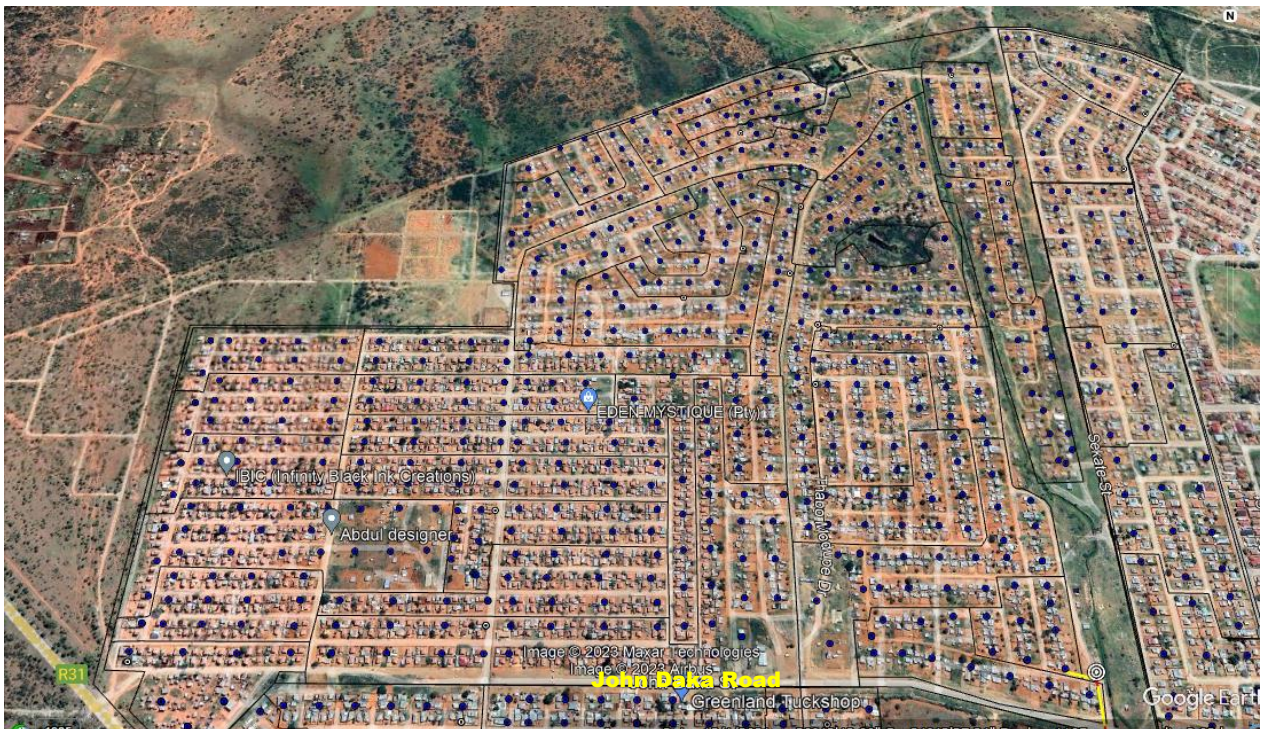
Figure 20: Section 1 of Route 1: John Daka Road and residential areas of Galeshewe to the north (the blue dots show the proposed position of the poles for the aerial fibre (either mid-block or on the pavement areas of the road reserve))
