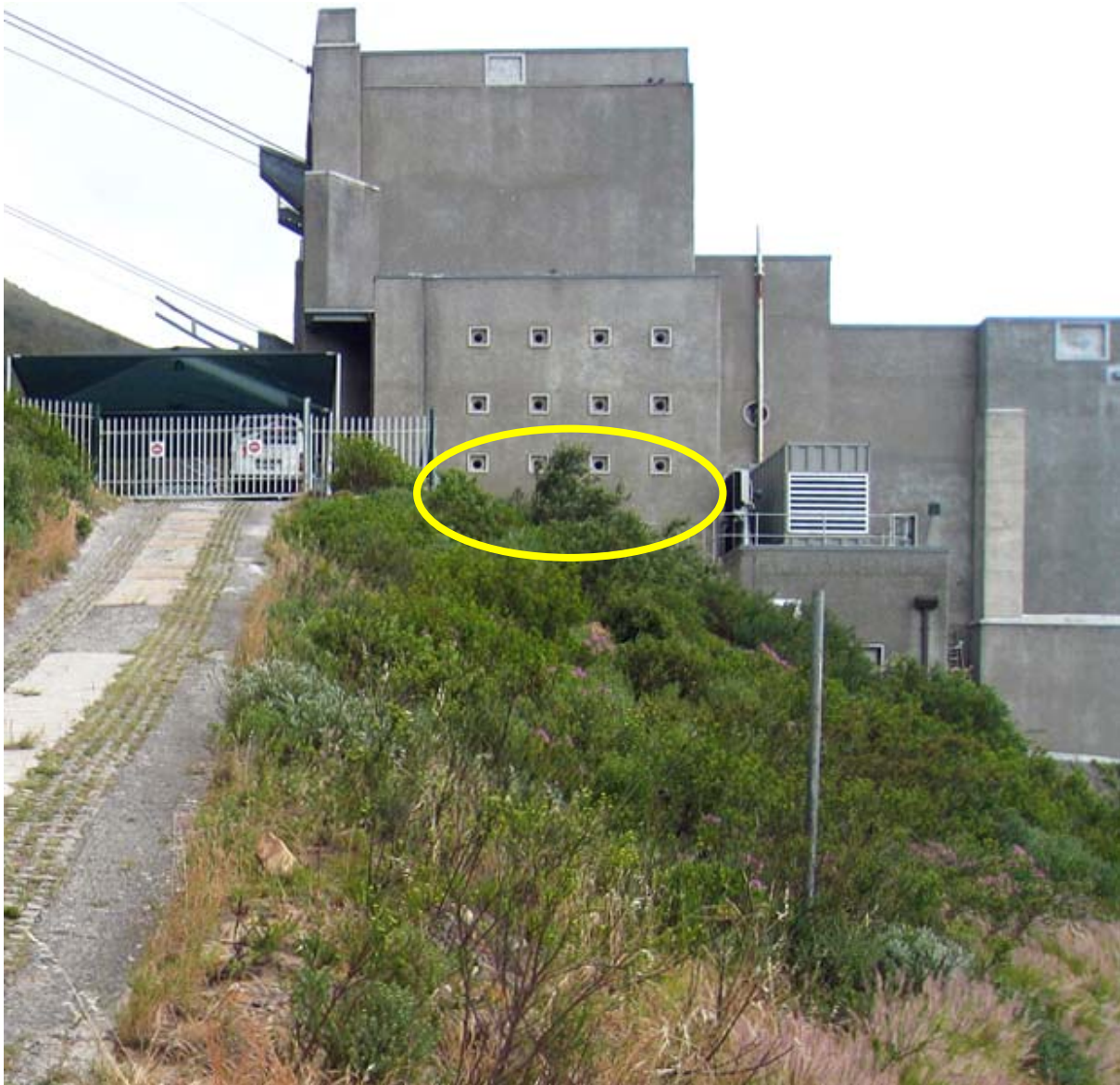
Lower Station from the east, with the location of the proposed canopy over the existing bridge circled in yellow.
