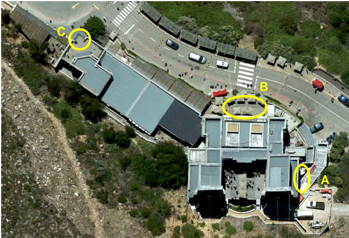
A 2015 aerial photo of Lower Station, with the three project sites circled in yellow. (Source: City of Cape Town)
