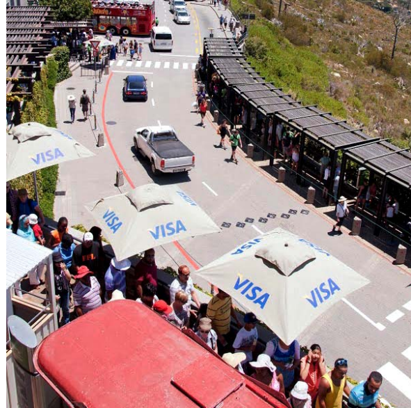
View of the Level 2 balcony from above, with visitors queuing in the sun before ascending to Level 3, where they will board the cable cars. The proposed pergola will have the same construction materials and finishing as the existing pergola structures.
