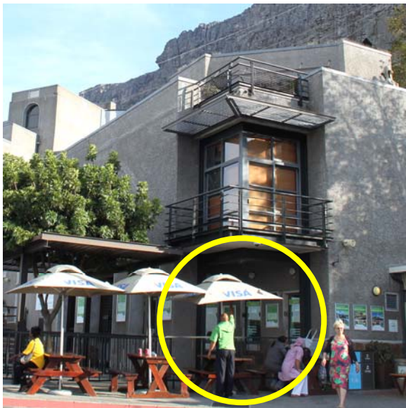
The corner of the Administration Wing, with the location of the recessed ticket office and kiosk circled in yellow on the left, with more detail shown on the right. The new corner door will align with the existing I-beam above.
