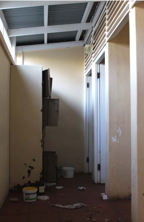
Interior of the building
