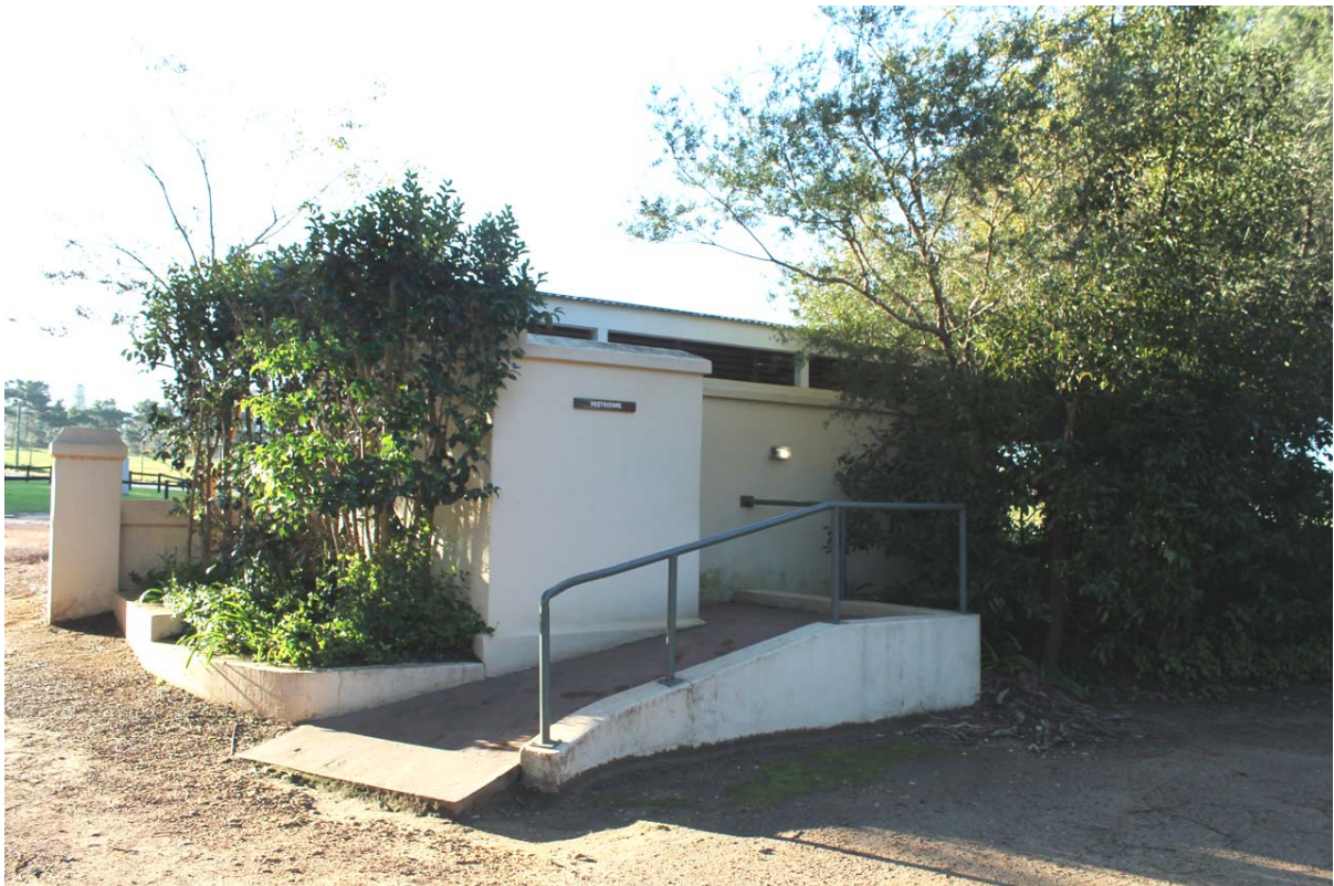
View from the south-west
