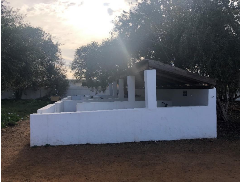
Figure 15: East elevation of 'pigsty' proposed to be demolished.
