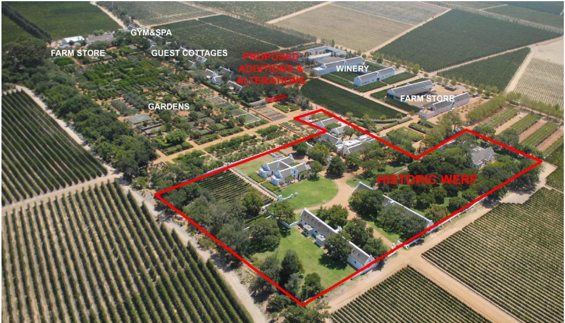
Figure 22: Aerial photograph showing the proposed development in relation to the historic werf.
