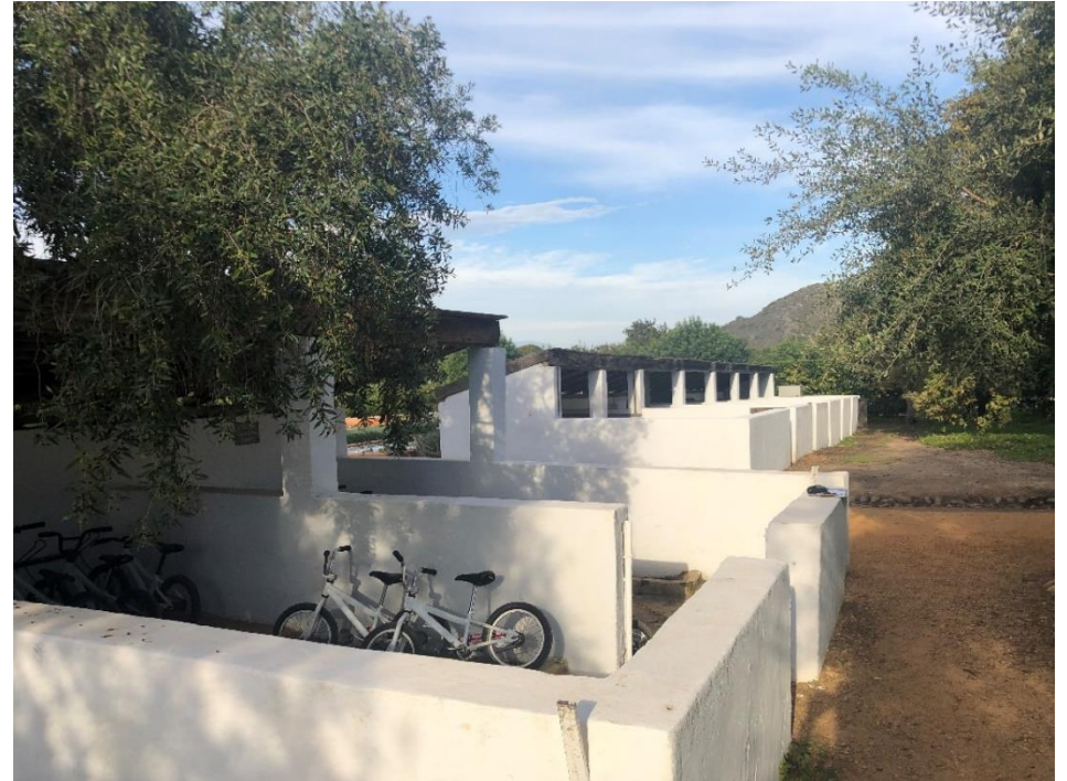
Figure 16: West elevation of 'pigsty' to be demolished in the foreground, and 'pigsty' to be altered seen beyond.
