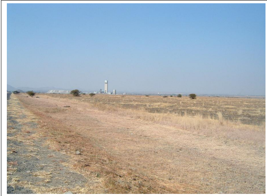
Figures 4 & 5- The expansion of the waste rock dump associated with Shaft 16 (in the background) will occur on a level stretch of land that is partly covered with grass veld and with agricultural fields (above and below).
