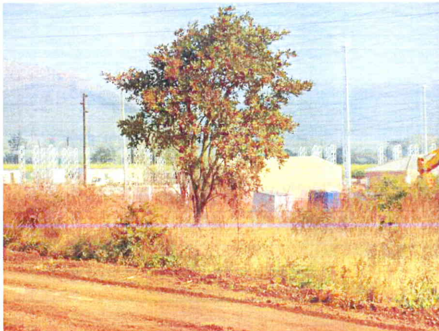
Figure 5 The Malelane substation where the proposed Khanyazwe Switching station will be erected.
