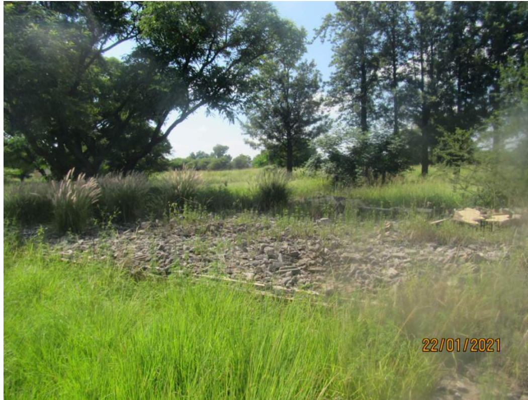
Figure 23 – Foundation located at WK003
