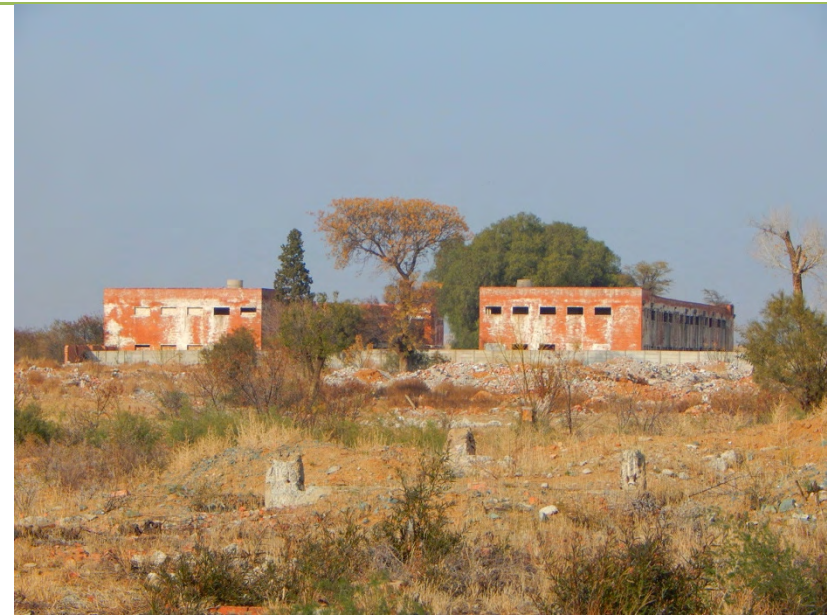
Figure 51: Rubble remains of a hospital (inside Shaft 1# area)
