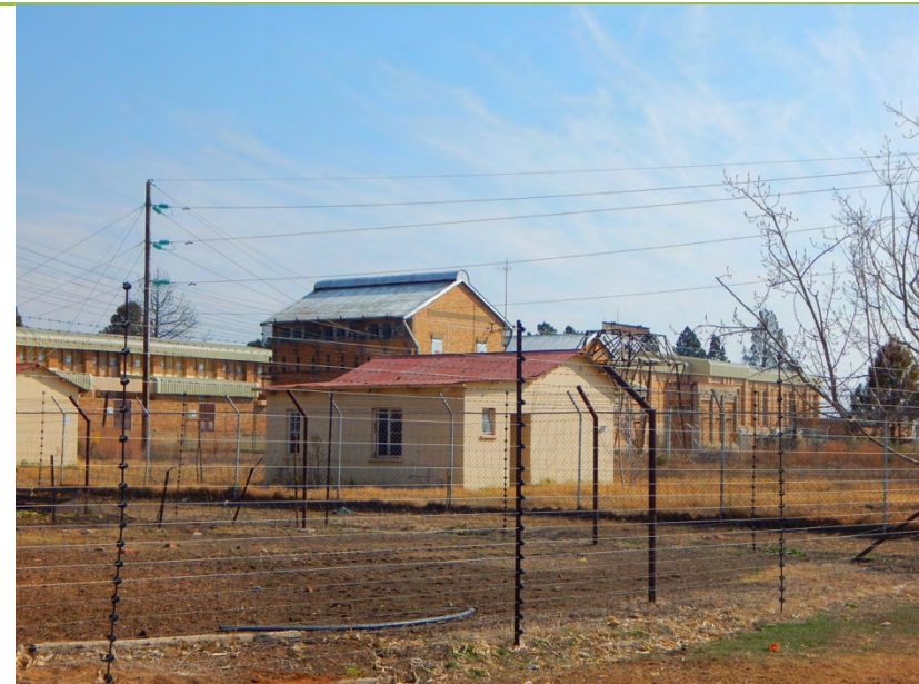
Figure 49: Water works structures (within lease area)
