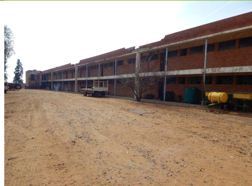
Figure 50: Historical hostel (inside Shaft 1# area)
