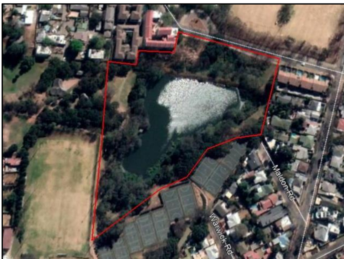
Figure 7. Aerial view of the dam location dating to 2020 (Image: Google Earth)
