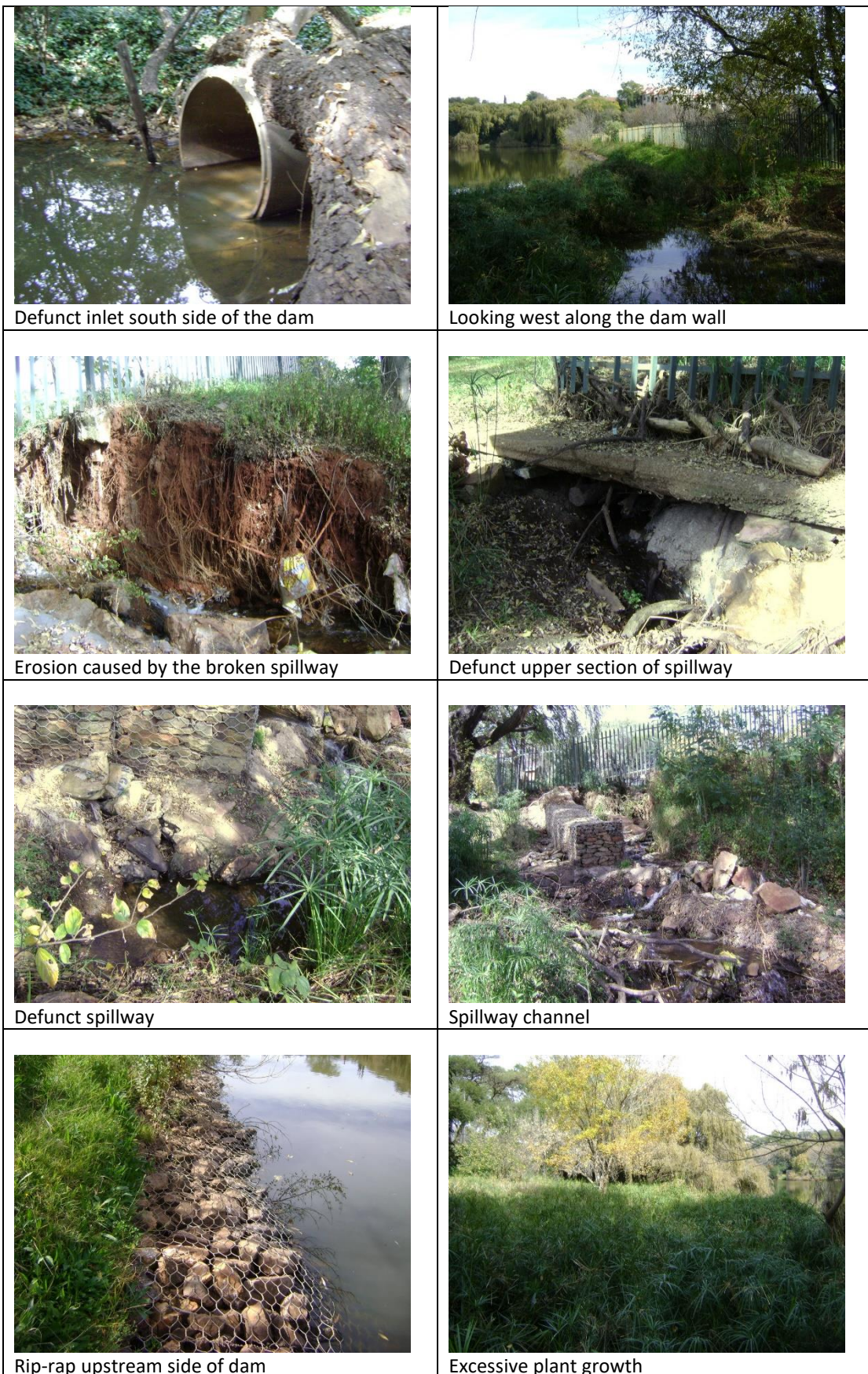
Figure 8. Various elements regarding the dam
