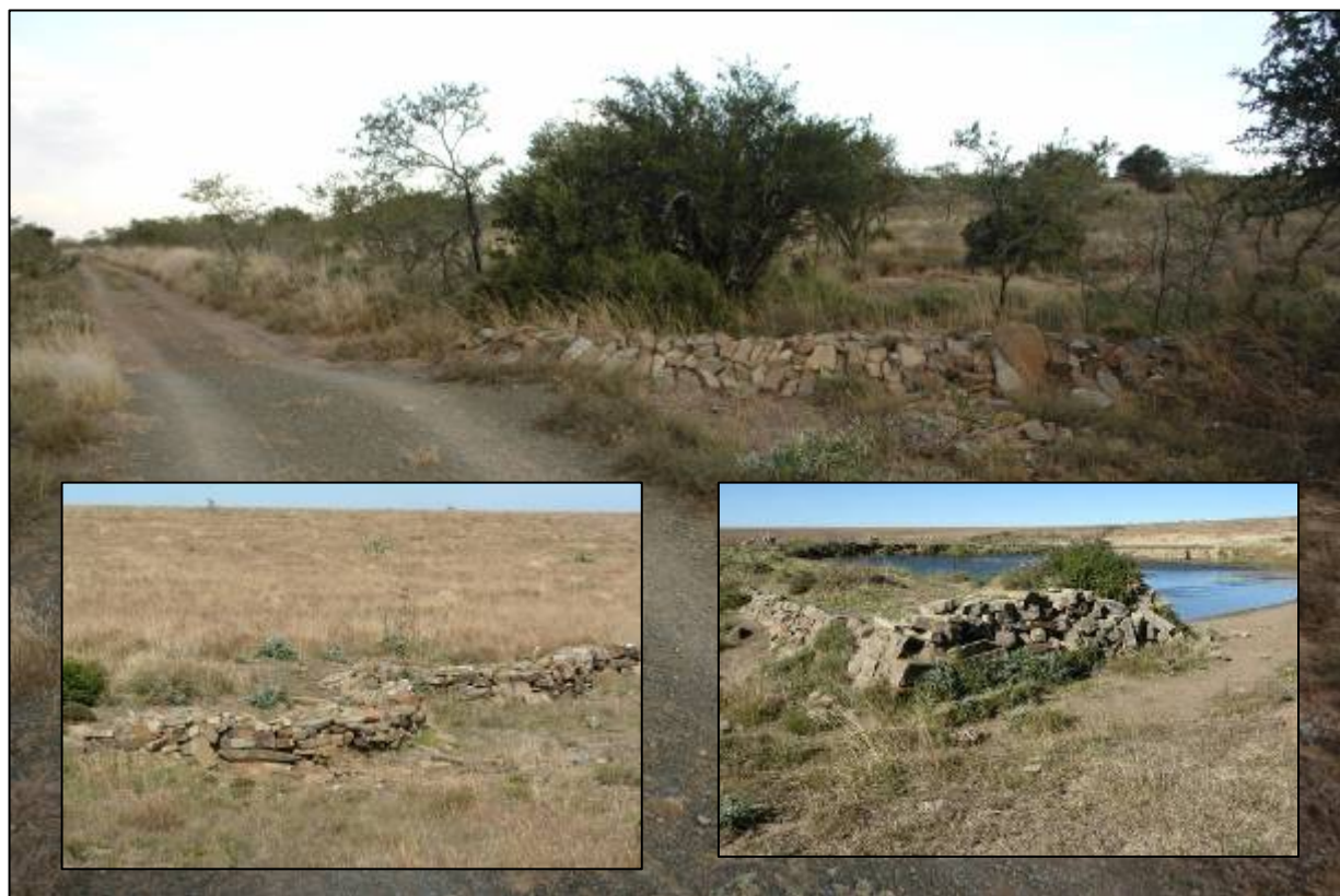
Fig 18. Examples of everyday functional use of stone, which include the construction of water furrows, dams and erosion prevention walls. These features are often changed/re-built and have little heritage value.
