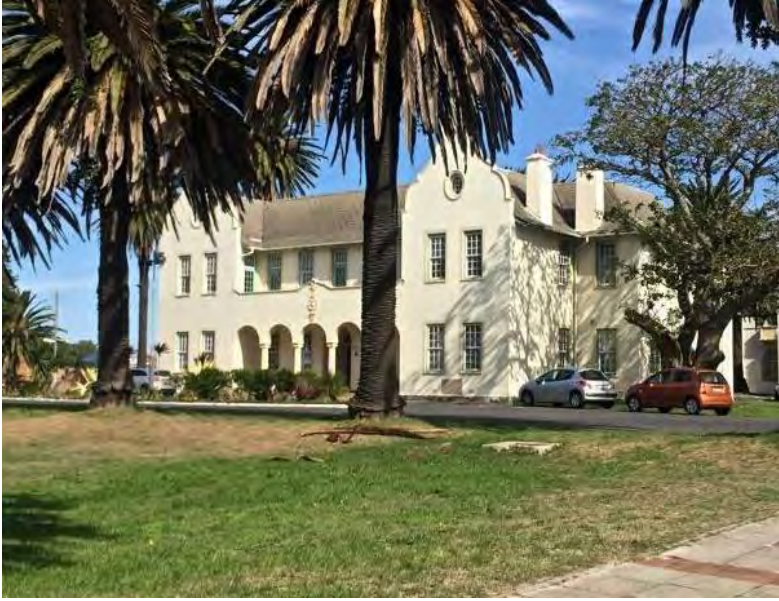
Fig 8.5. The Administration Building Alexandra Institute
