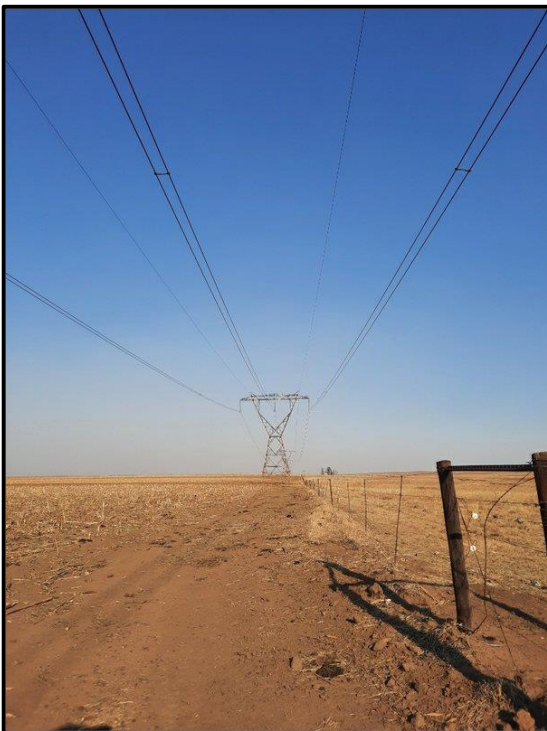
Figure 7.3. Existing powerline next to cultivated area.
