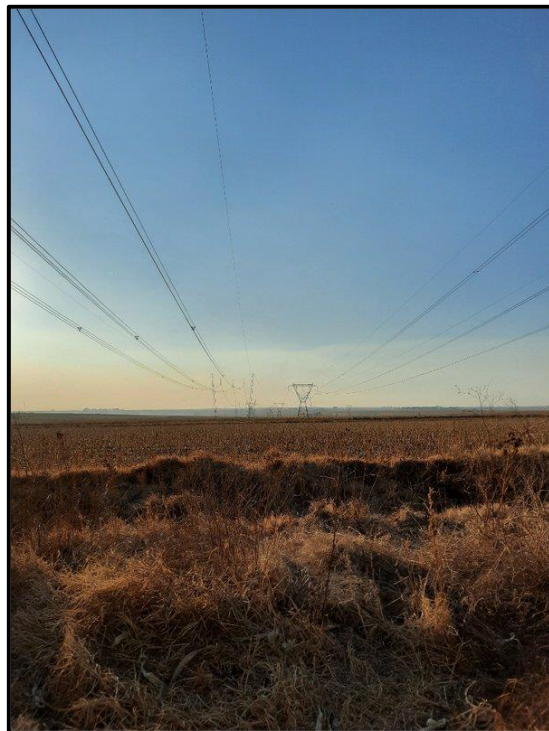
Figure 7.4. General site conditions under existing powerlines.
