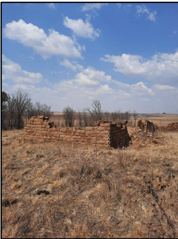
Figure 8.4 Sandstone walls at Waypoint 074.
