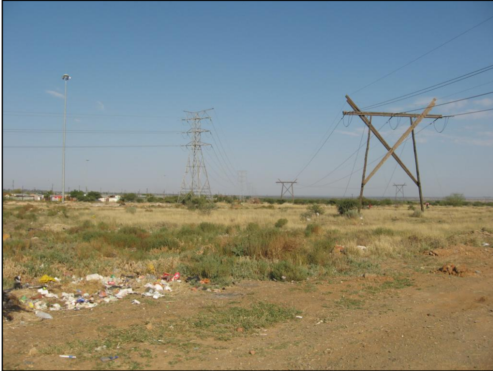
Figure 7: Alignments of PV3 closer to Kimberley.
