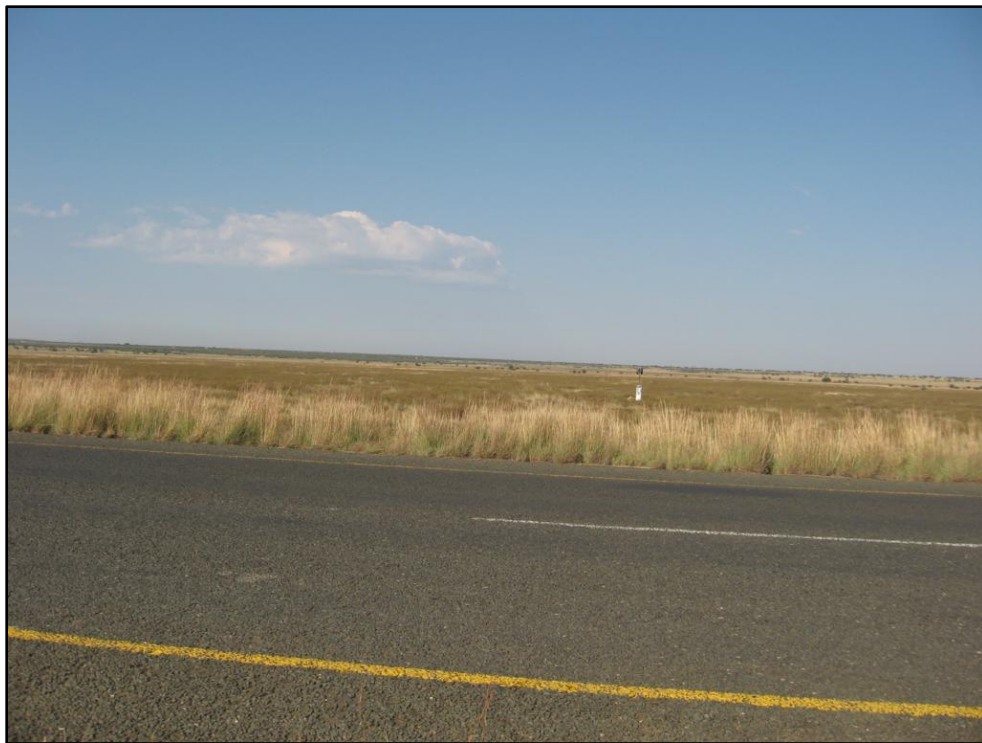
Figure 8: Crossing point of one of the alternative lines on N12
