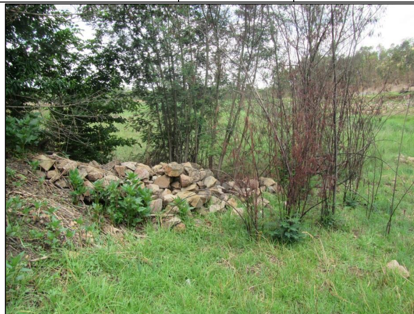
Figure 26 – Alternate view of the interior of portion of the stone walling
