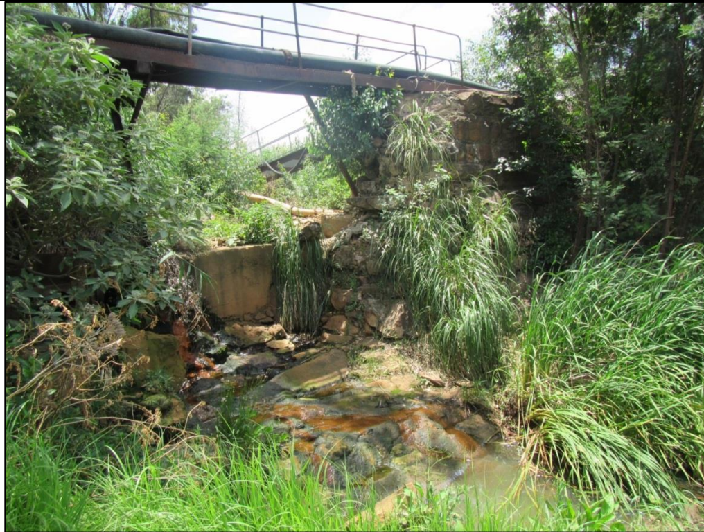
Figure 24 – View of Rosherville Dam spillway
