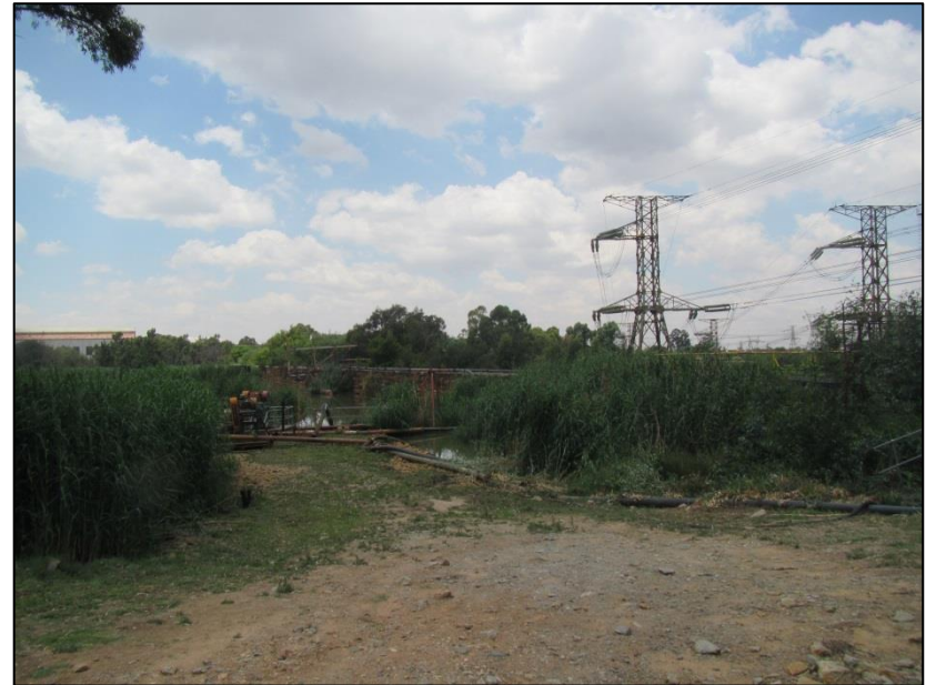
Figure 23 – View of inner side of dam wall
