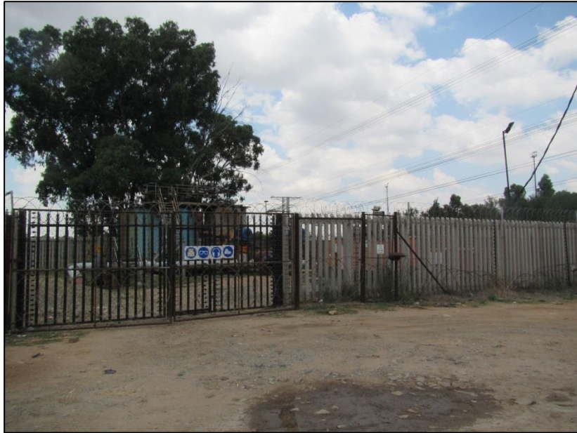
Figure 22 – View of pumping station at western end of dam wall that is still in operation
