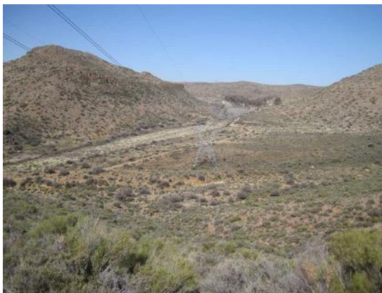
Figure 14: View of one of the power lien corridors
