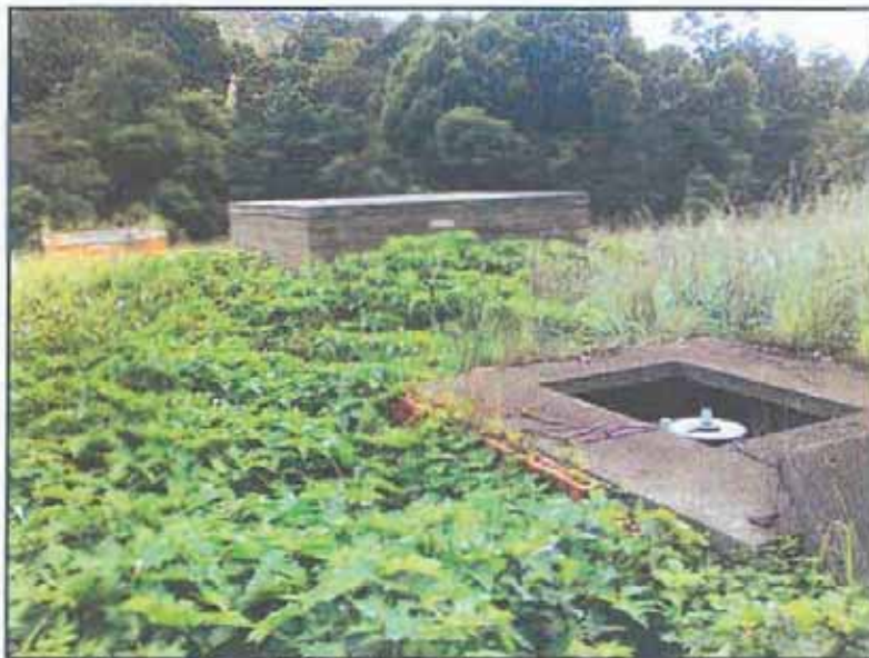
Figure 4: A water pipeline runs through the valley region.
