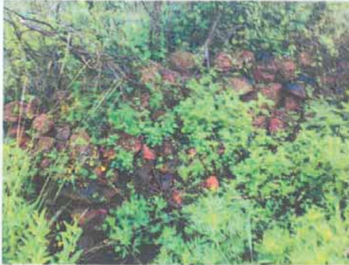
Figure 30: A section of the stone wall.
