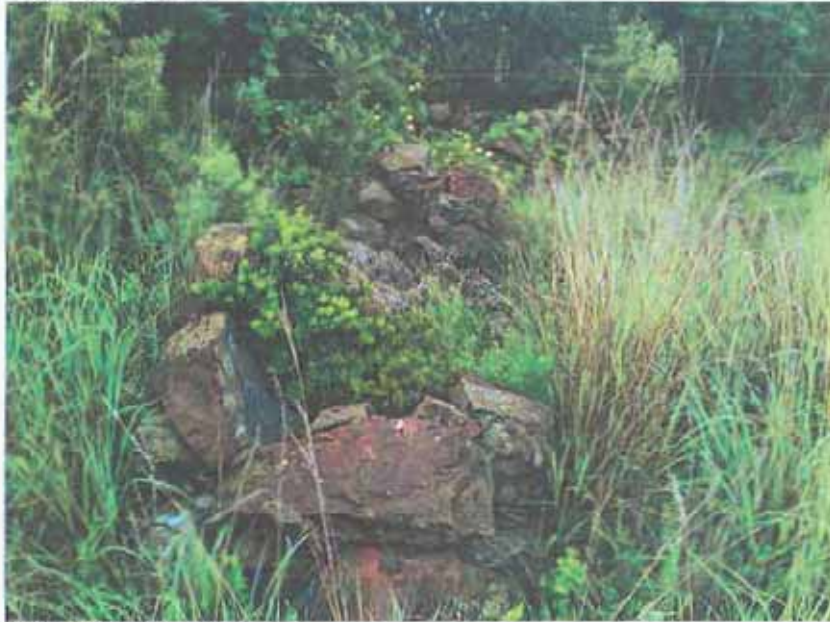
Figure 35: A section of the stone wall.
