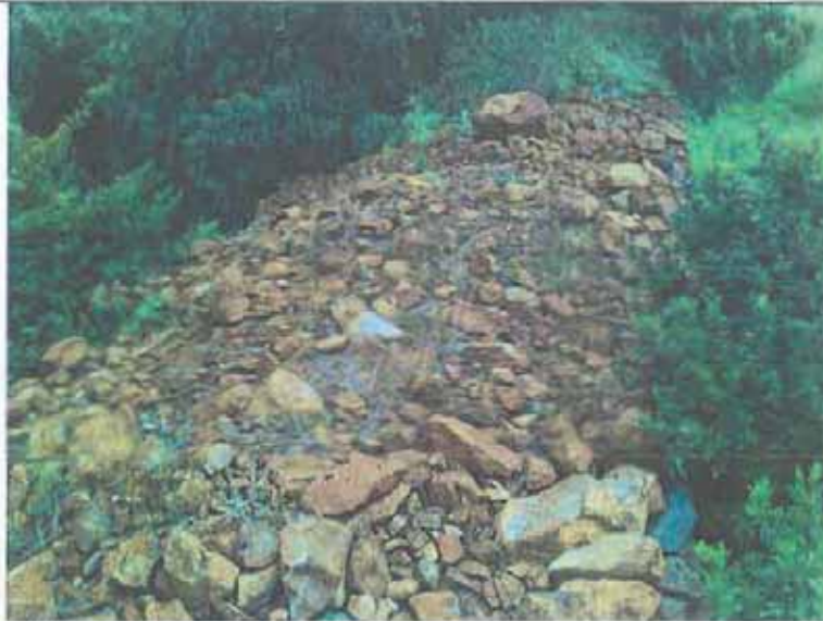
Figure 18: Stone walling as part of terracing.
