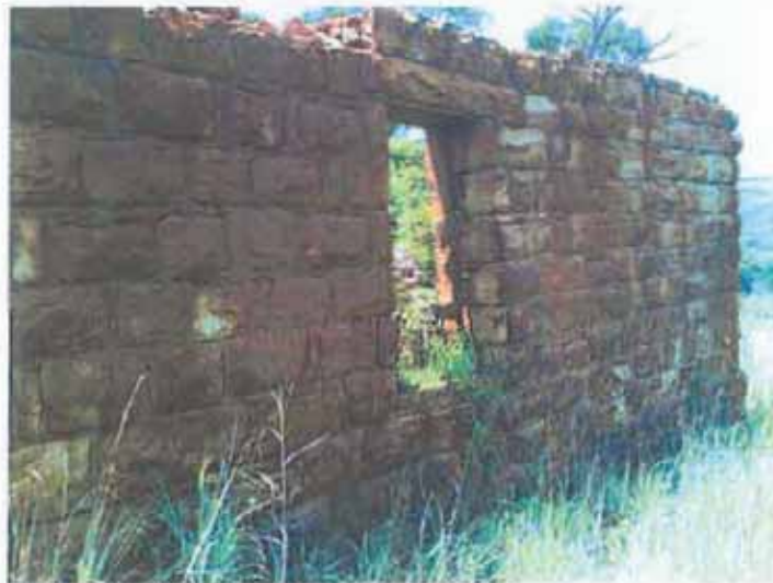
Figure 14: The dressed stone and lintel are clearly visible.
