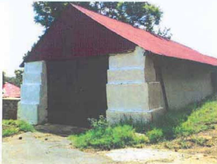
Figure 28: The western entrance of the main farm shed.
