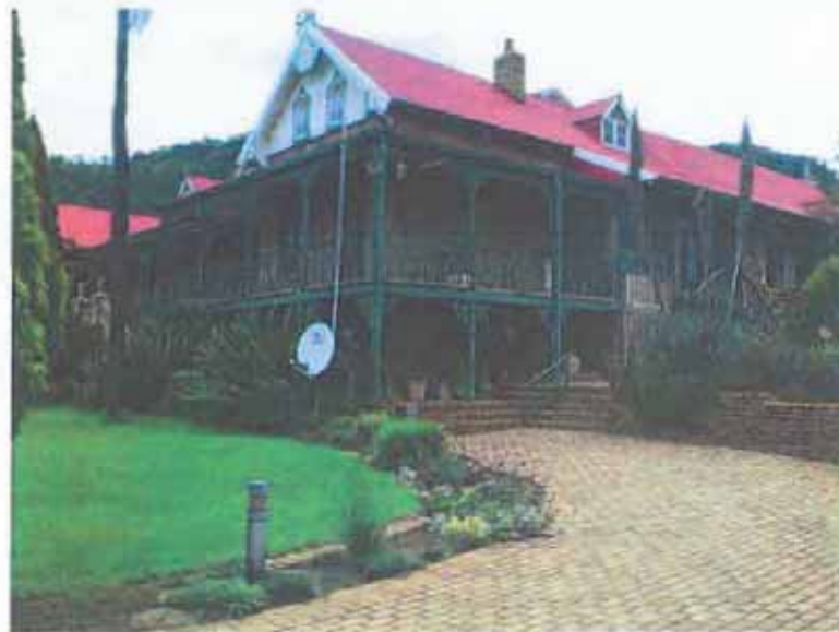
Figure 22: The eastern façade of the main house.
