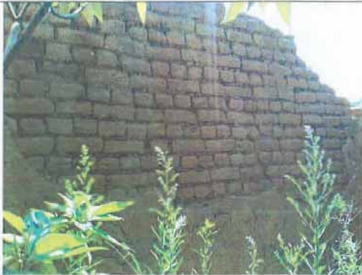
Figure 13: Sun dried mud bricks were used to subdivide the rooms.
