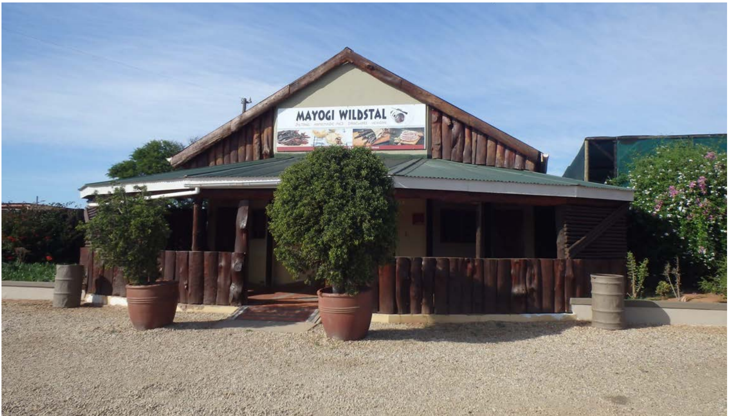
Figure 4.1: Existing structures located in the south east of the property
