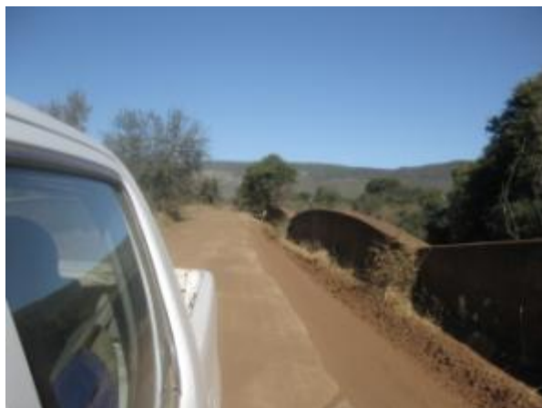
Fig. 35. The bridge and its older predecessor, a weir, in this same area should be protected if new roads are considered. (Photograph S.M. Miller 2011)
