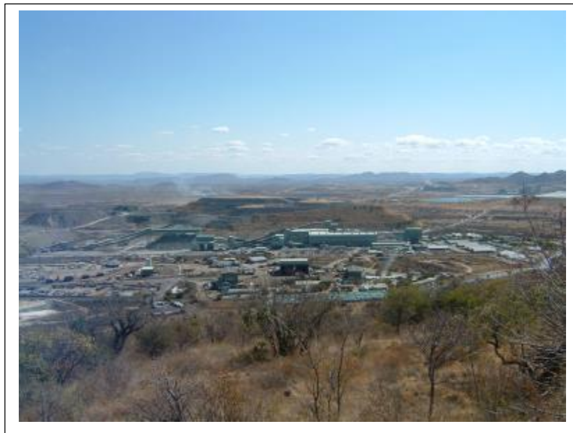
Figure 2- The proposed Akanani Substation is located behind the waste rock dumps in the south-eastern corner of the farm Zwartfontein 814 (above).
