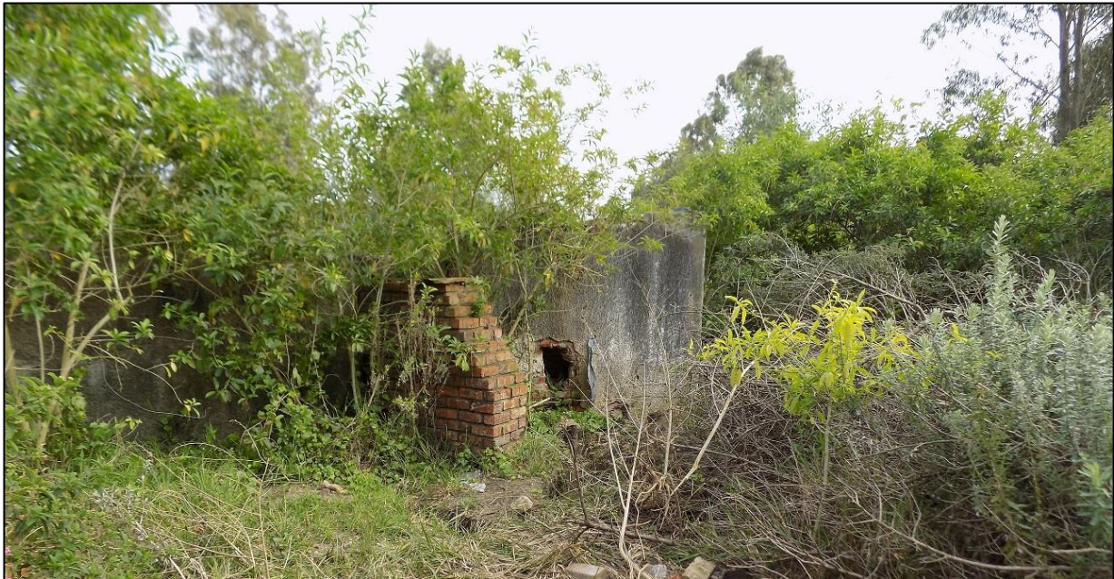
Figure 1. General views of some of the structures located within the proposed development area on on Erf 7005 Portion of Erf 1935 in Walmer, Gqeberha (Port Elizabeth), Nelson Mandela Bay Municipality, Eastern Cape Province.
