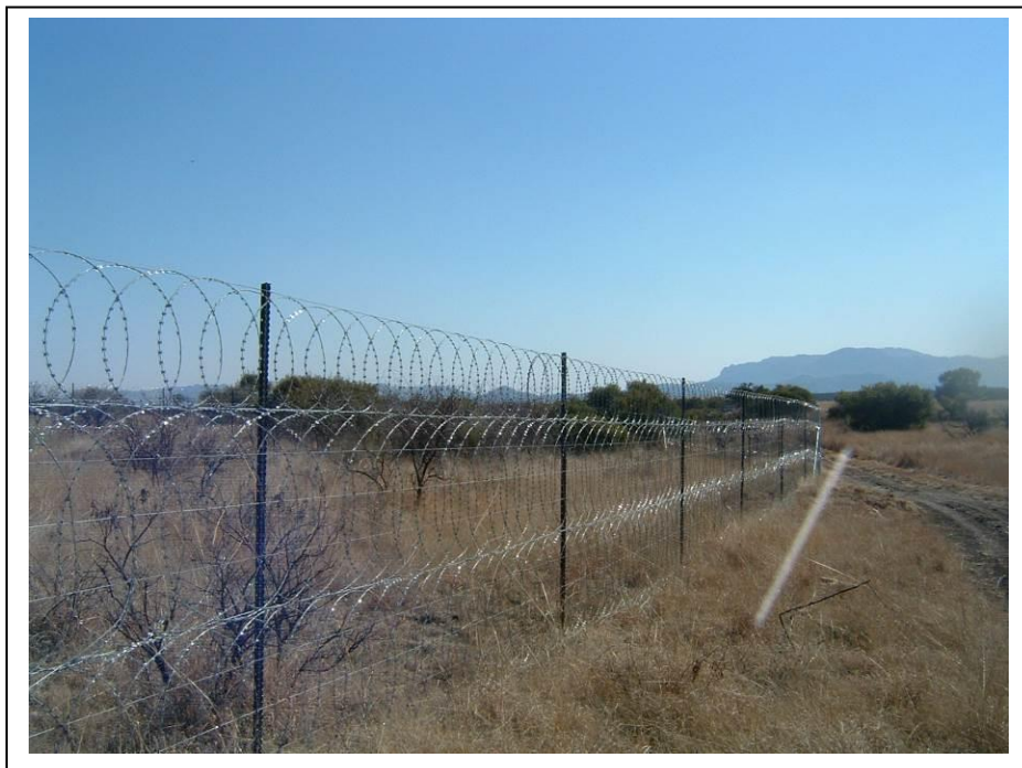
Figure 12- GY02 is located on the western perimeter of Heric Bokfontein's border and outside the mine's jurisdiction (above).
