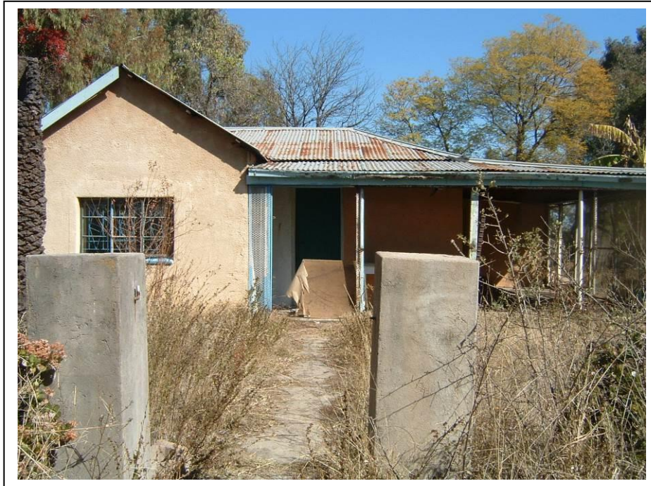
Figure 13- A historical house (HH01) near the western border of the Bokfontein Chrome Mine (below).
