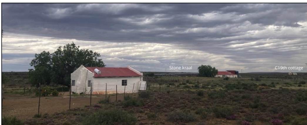
Figure 26: Cottages and kraal associated with Trakaskuilen farmstead.
