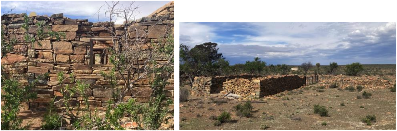
Figure 45: Stone farm house dry packed wall and dry stone packed kraal structure associated with dam on Witpoortje farm.
