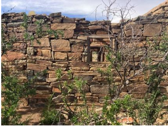
Figure 45: Stone farm house dry packed wall and dry stone packed kraal structure associated with dam on Witpoortje farm.
