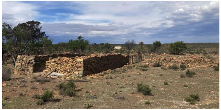
Figure 45: Stone farm house dry packed wall and dry stone packed kraal structure associated with dam on Witpoortje farm.
