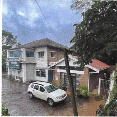
BUILDING 2 (out-building) North - West Elevation
