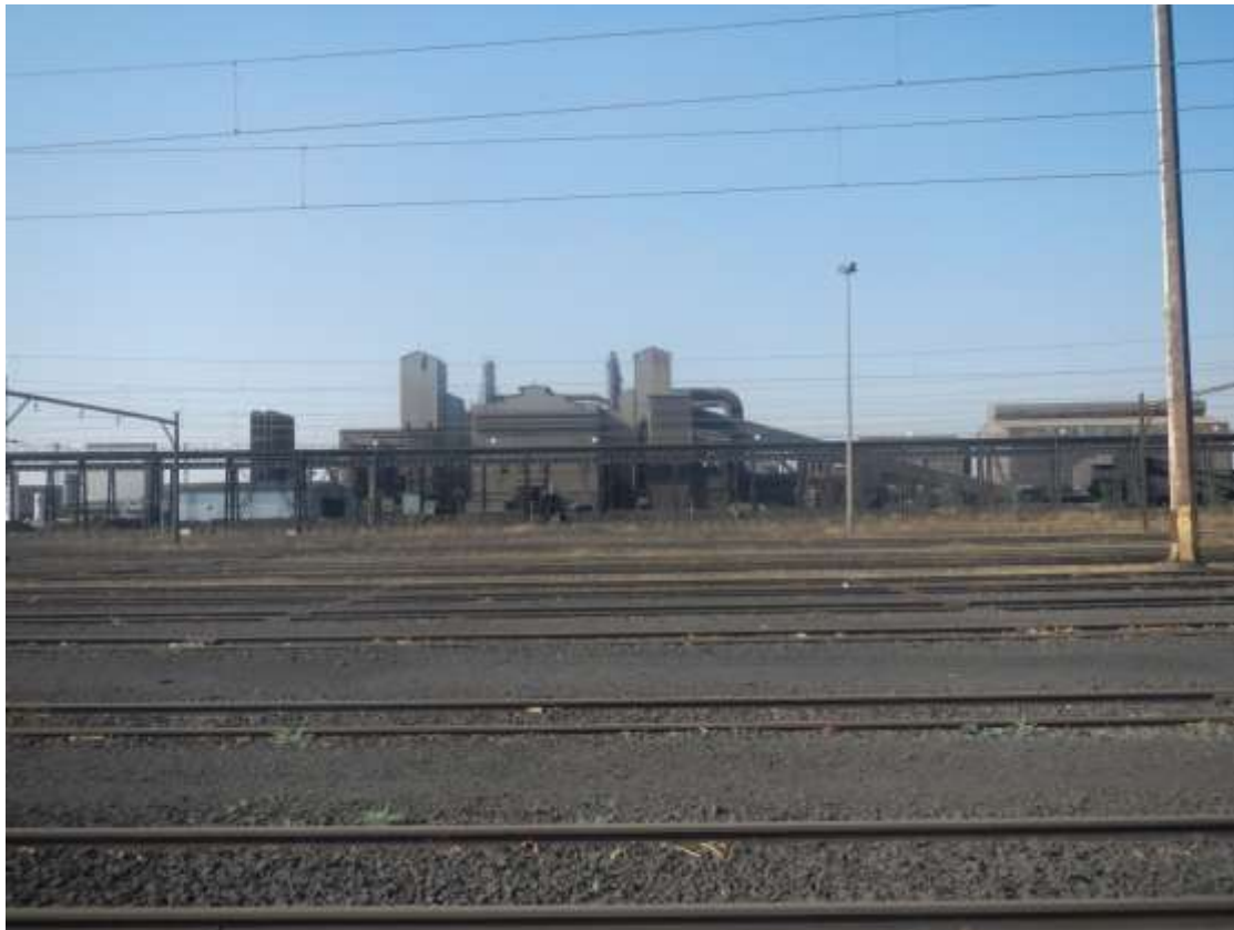
Figure 7: A view of Trans Alloys a coal dependent industry close to the Marshalling Yard
