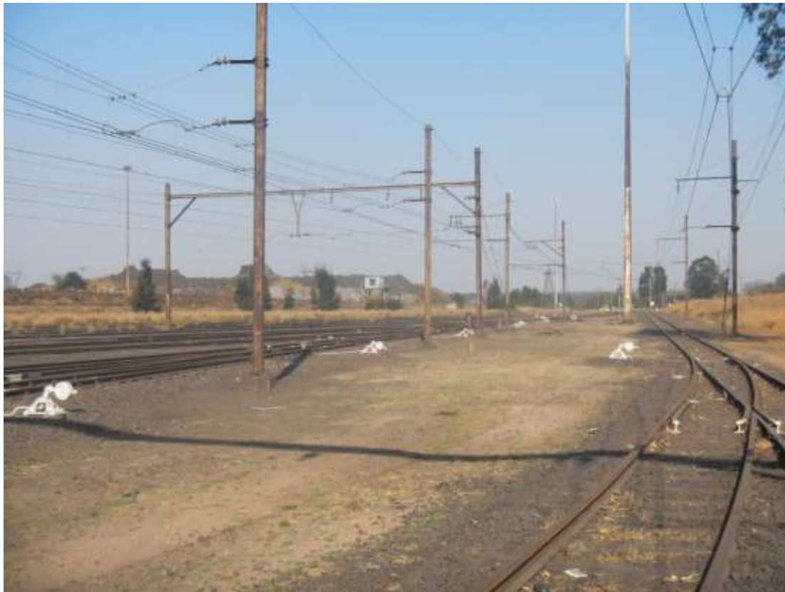
Figure 5: View of the southern end of the proposed project area
