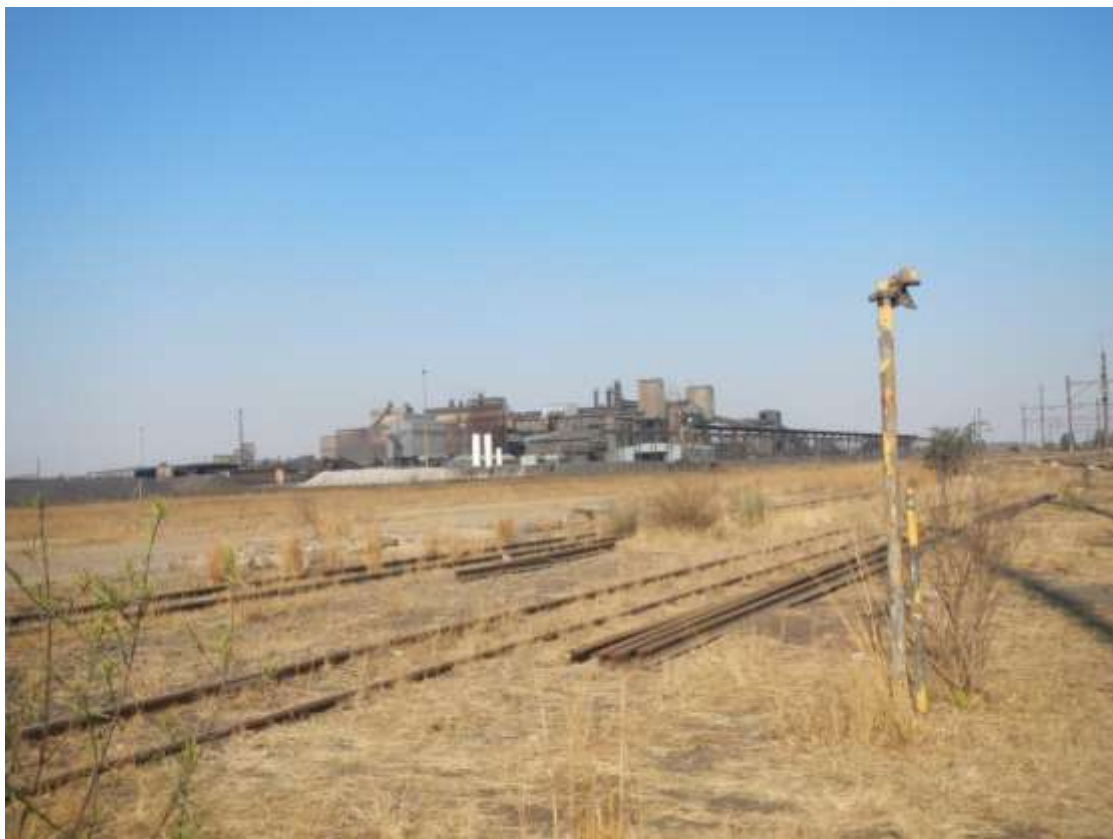
Figure 8: View of the Trans Alloys from the south -western side of the study area
