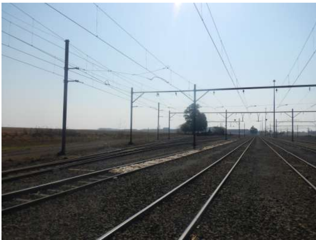
Figure 10: Part of the railway line on site
