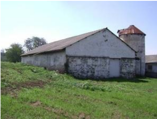
Figs 5 and 6: The covered space between shale barns and Barn no 1 with a silo behind
