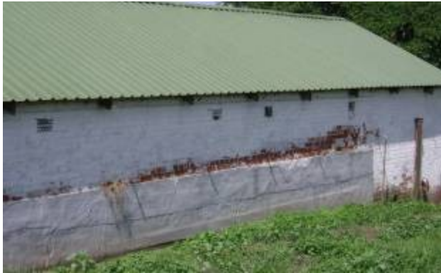
Figs 7 and 8: Showing the old brick barn: the portion towards the trees is in English bond suggesting that this portion was pre- or immediately post- World War II.
