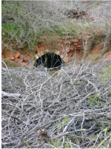
Entrance to overgrown brick kiln S33 45 279; E25 39 721 (Photo JS Bennie)
