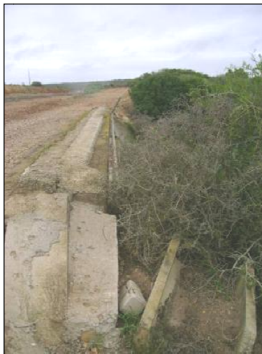
Old Railway Bridge (Photo: JS Bennie)
