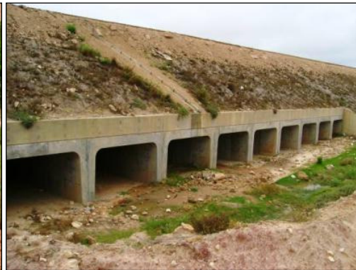
Culverts—old on left, new (2009) on right S 33 45.311; E25 39.445 (Photo: JS Bennie)
