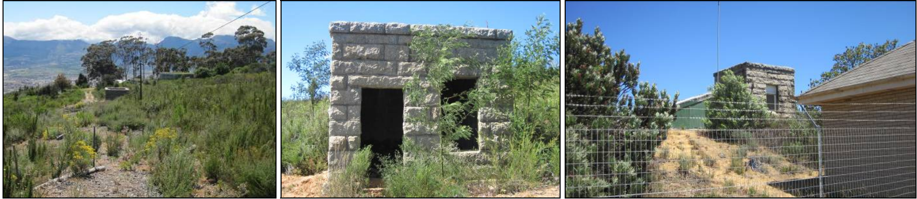
Plate 1: View towards the Meulwater WTW with a small structure built of granite in the foreground. The small building may have served as a pump station/valve house and still lies over an in use pipeline (though not affected by the current upgrade). Plate 2: The north face of the granite building. Plate 3: A structure of similar dimension and style encapsulated within the Klipdam Reservoir precinct.
