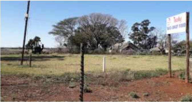
View of the farmstead from the North boundary
