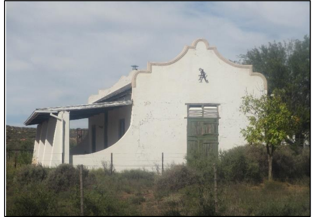
Figure 81: The stable manager's house at waypoint 1552 in HL03.
