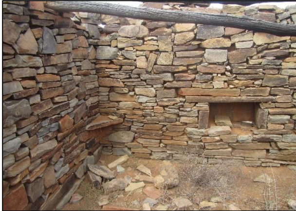
Figure 46: Architectural details in the ruin at waypoint 185 in HL03.
