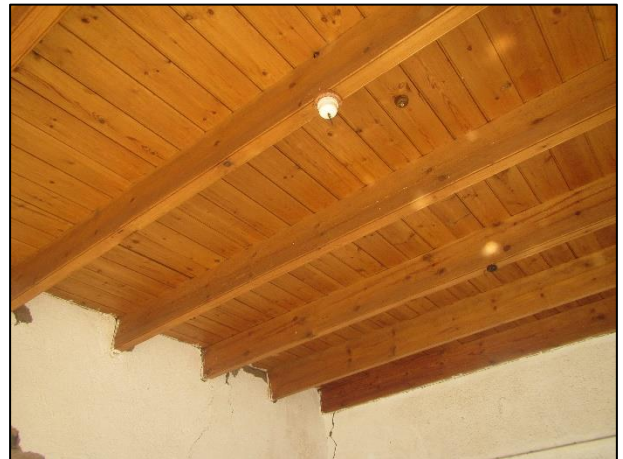
Figure 87: An intact ceiling in the main house at waypoint 1791 in HL04.
