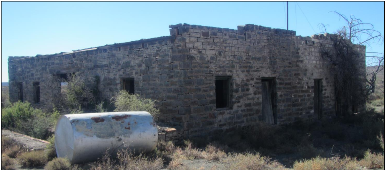
Figure 88: A derelict outbuilding alongside the main house at waypoint 1791 in HL04.
