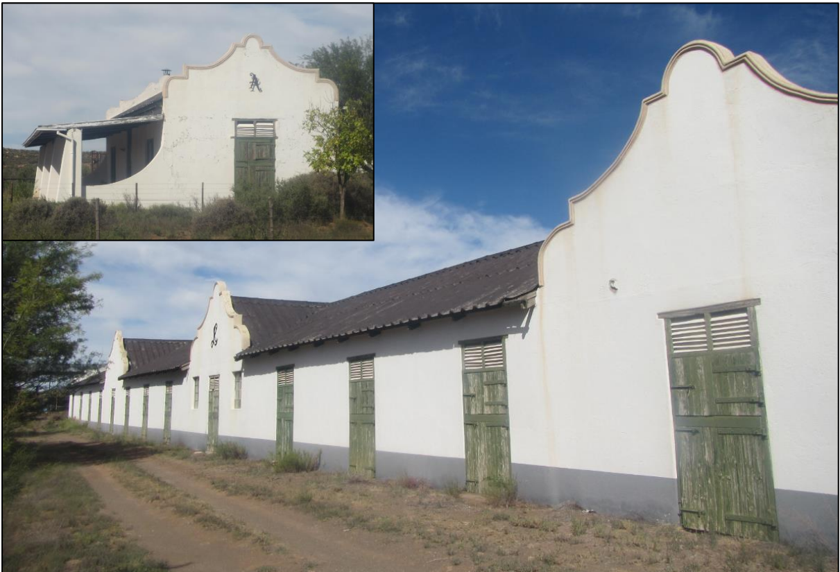
Figure 13: Disused stable building with stable manager's house at waypoint 1552.
