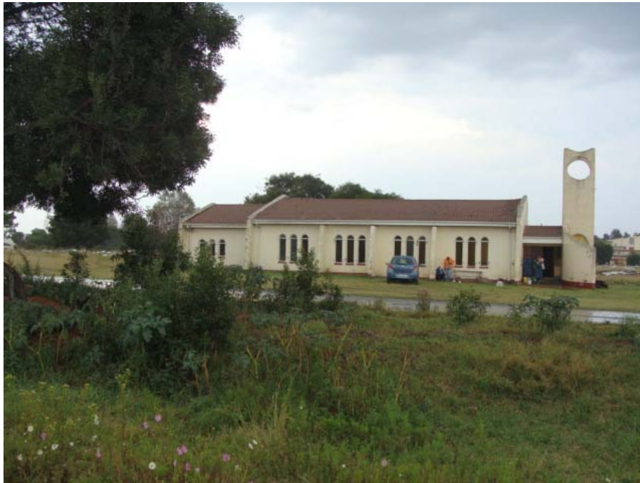
Figure 17: The church at the demolished New Town Village.
