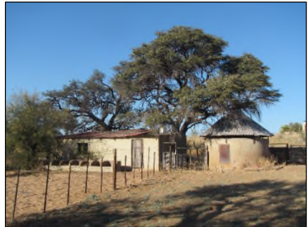
Figure 41: Outbuildings at waypoint 1162.
